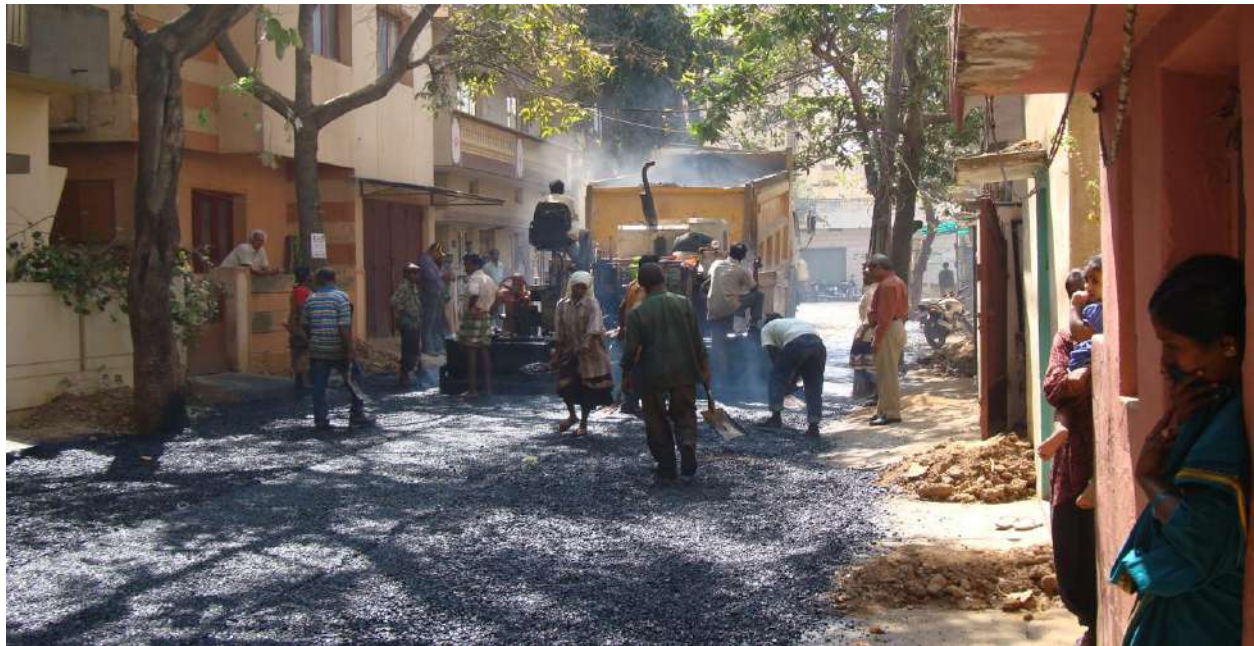
Figure-3.6: Asphalt paving process in the study area
