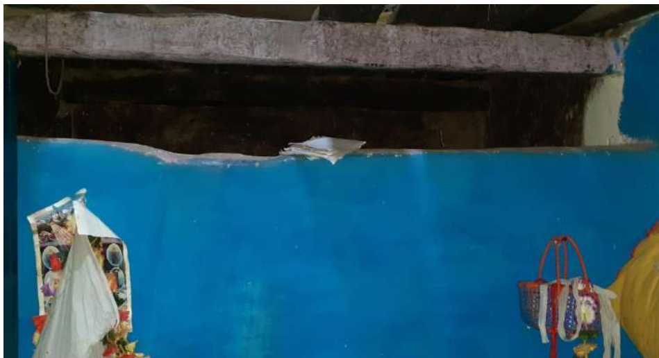
Figure 5.1. Panatha of Cement and Brick made open top like structure.
