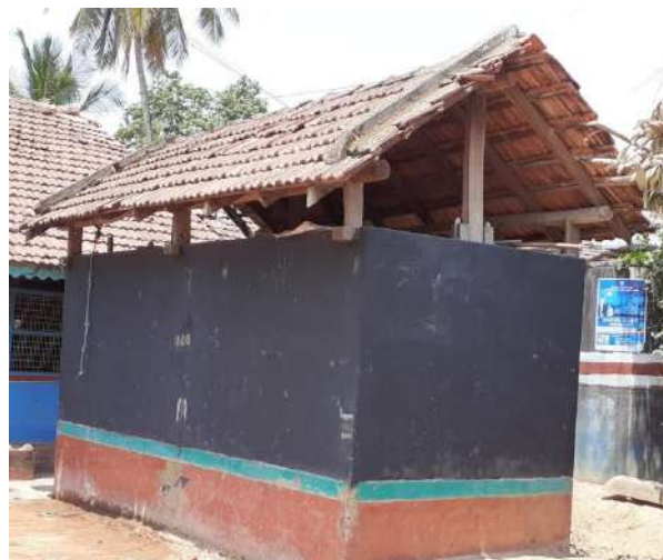
Figure 5.4 Panatha structure made of Cement and Brick top closed
