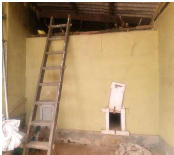
Figure 5.3. Panatha structure made of Cement and Brick provided with opening at bottom to unload.
