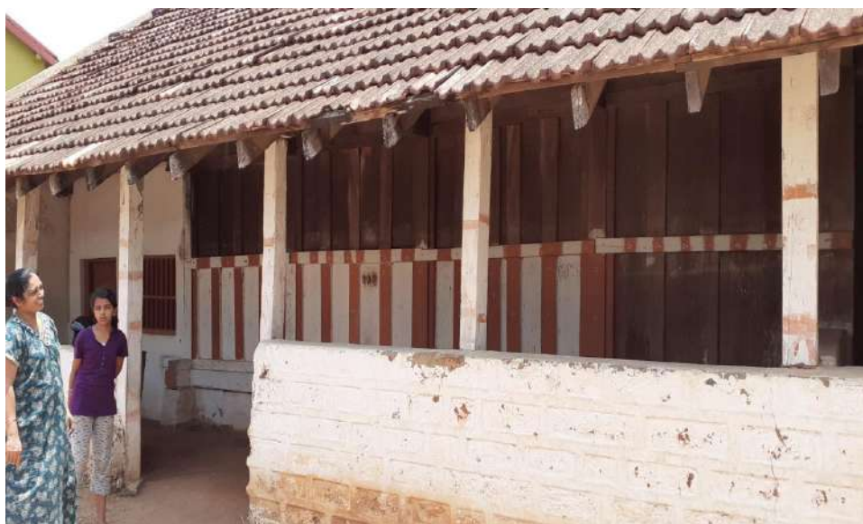
Fig. 4.2 Panatha made of wood six chambered structure.
